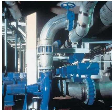
**A resilient seated butterfly valve with superior design features and materials of construction to provide repeatable tight shutoff in severe abrasive and corrosive environments for a variety of applications.**
