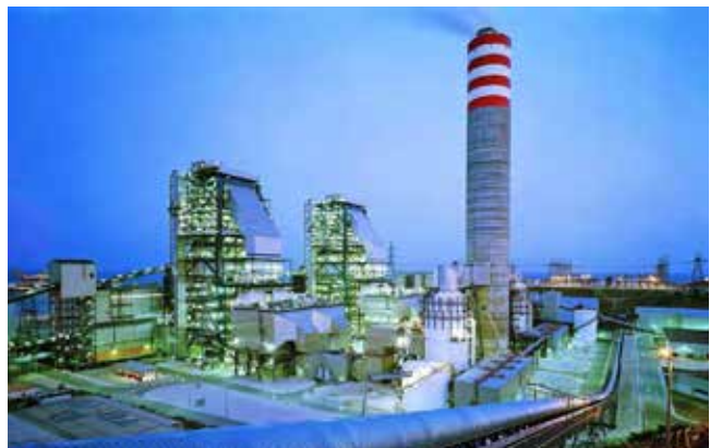
Power Plant Iskenderun, Seawater FDG (Turkey)
