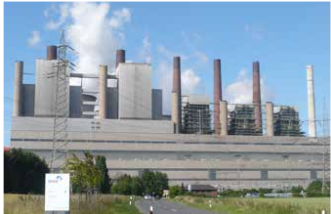
Power Plant Neurath (Germany)
